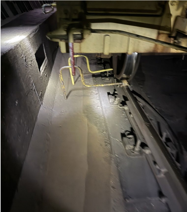
Photo 3: Shows the proper placement of wheel chocks to prevent any unintended movement on the work flat.
