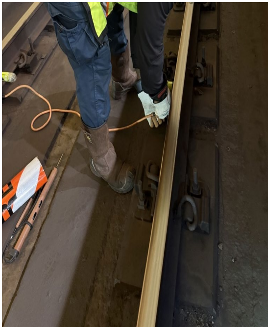
Photo 4 (left): Shows RWIC installing shunts using the required Class O insulated gloves. Photo 5 (right): Compliant Class O insulated glove.
