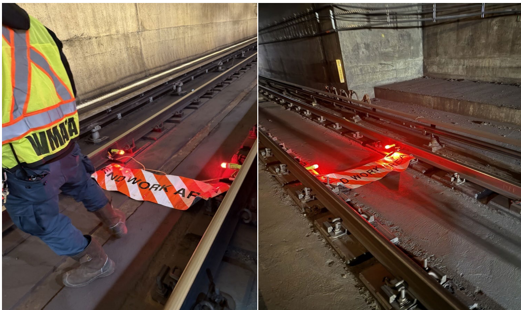
Photo 5 (left) and Photo 6 (right): Shows the correct placement of the shunting devices accompanied by two (2) red lanterns or e-flares, and “End Work Area” mats.
