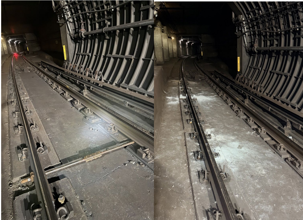
Photo 1 (Left): Fastener location with a gauge rod present to hold the standard gauge at D2 045+10. Photo 2 (Right): Area after work was completed, and the gauge rod was removed.
