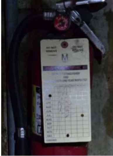
Photo 1 (left) extinguisher due for an inspection. Photo 2 (right) a loose extinguisher on the floor and not affixed to the wall.
