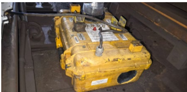
Photo 10: Properly installed WSAD.
