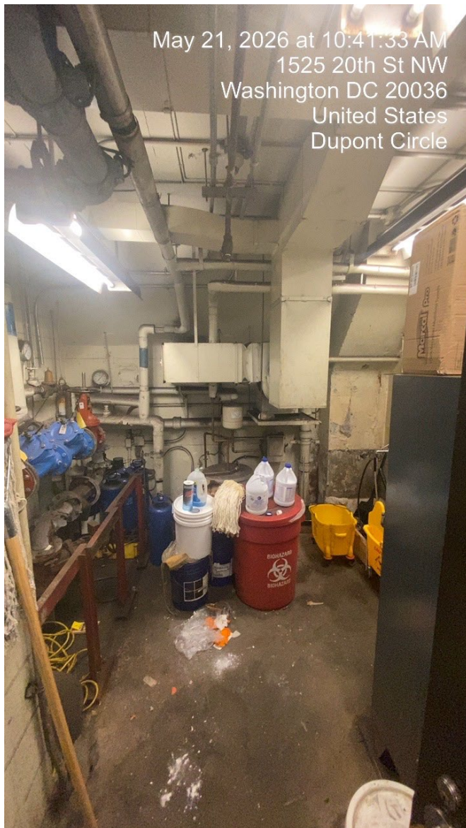
Picture 11 – Depicts interior view of Cleaners Room 204.
